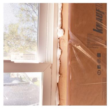
If you accidentally get out of control, like I did, don't worry! Allow the foam to dry (in about 4 hours) and you can easily cut away the excess foam with an exacto knife or box cutter.
