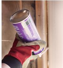
We decided to turn our one car attached garage into a room, so we installed two windows in the place where the garage door was. Our new wall has been insulated, and now it is time to insulate around the windows. We used DAP's No Warp Window & Door Sealant, according to directions listed on the canister.
